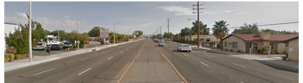
Sample of our 6 lane roads
