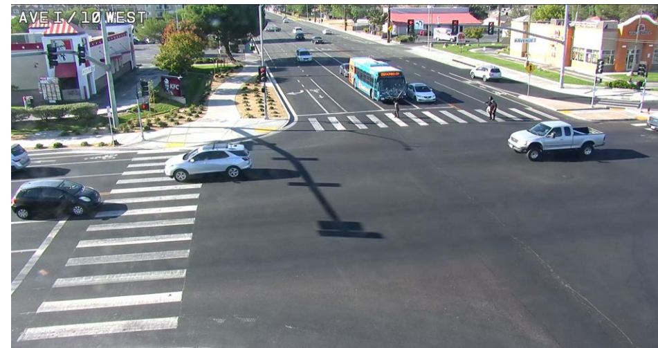
High Visibility Crosswalks & Curb Radii Reduction
