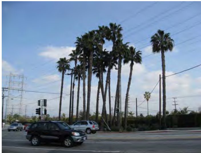
Cluster of Palm and high tension power poles at Fairfax Ave and La Cienega Blvd.
