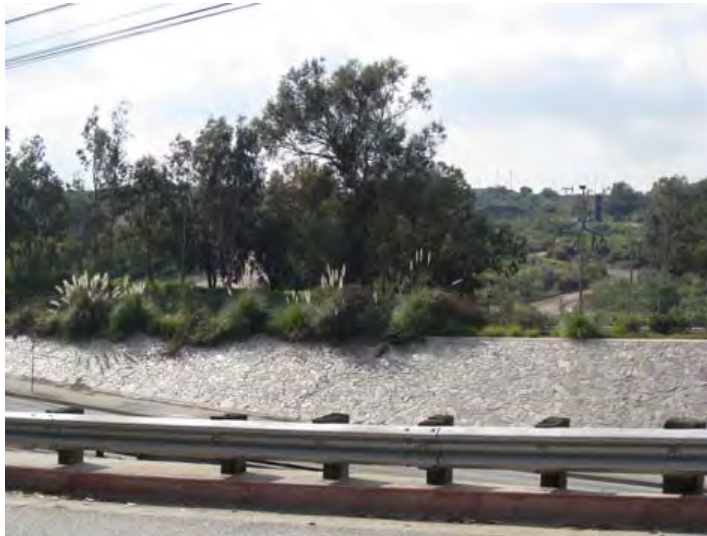
Embankment at Kenneth Hahn State Recreation area paved with flagstone & high-quality landscaping.
