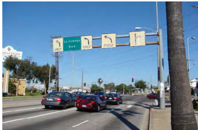
Three eastbound left turn lanes at La Cienega Boulevard and La Tijera Boulevard.
