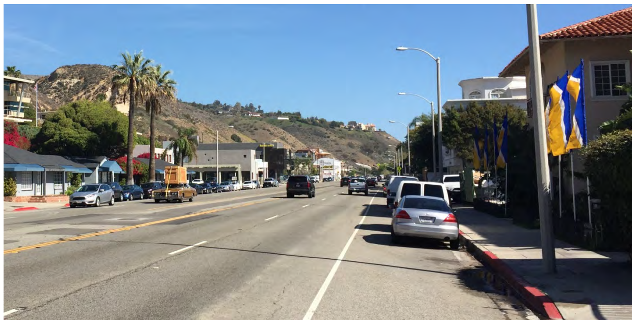
Figure 3-15 Red Curbs Improving Sight Distances around Driveways in Malibu Civic Center/Pier Area
